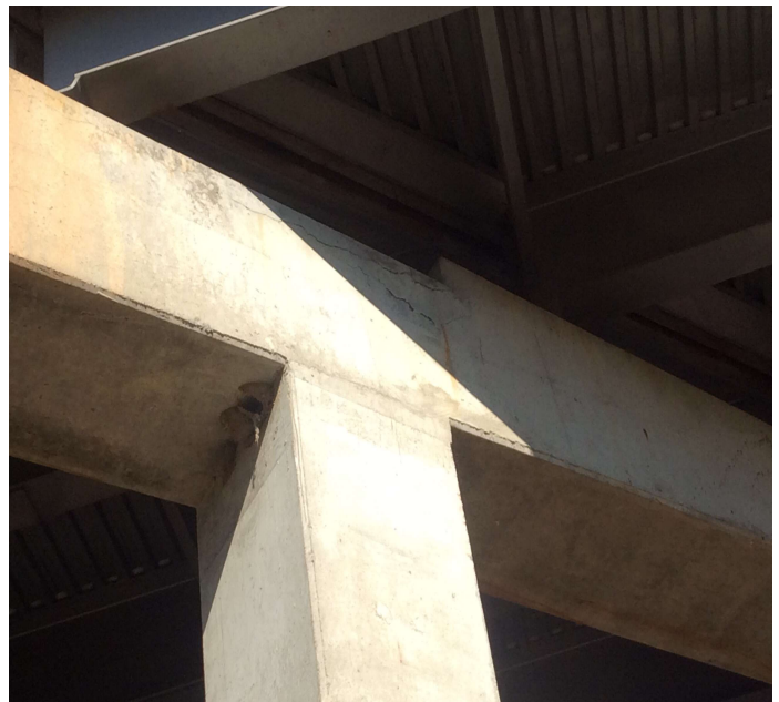
PHOTO 2 Description Bent #4 cap ahead face at column #3 transverse cracks (4'in length)
