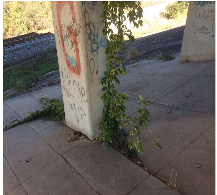
PHOTO 2 Description Tree growing up in slope pavement abutment #2
