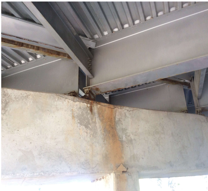
PHOTO 1 Description Bent #5 cap ahead face 4' transverse crack at top over column #2
