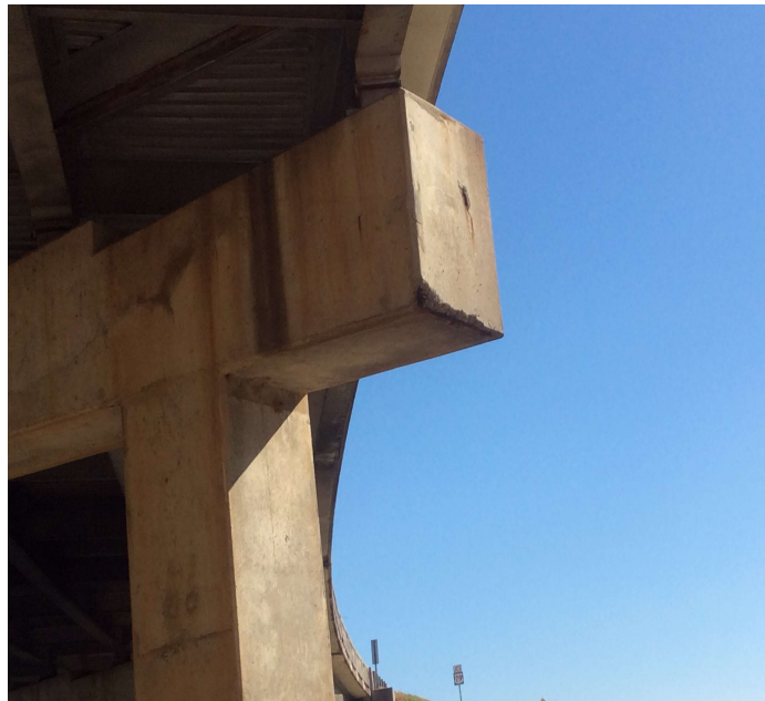
PHOTO 3 Description Bent #3 cap right end spalled with exposed rebar
