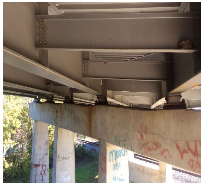
PHOTO 2 Description Span #1 bent #2 girders #2,3,5 have anchor bolts broken off
