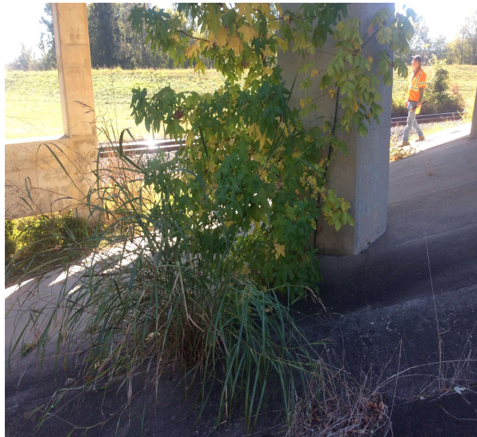
PHOTO 1 Description Abutment #1 trees growing up in slope pavement
