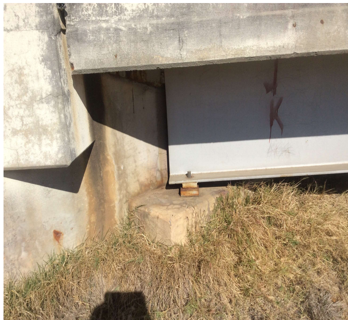
PHOTO 1 Description Bent #1 girder #6 outside anchor bolt nut missing
